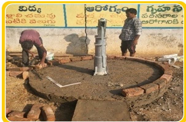
Platform & Soak pit Construction
